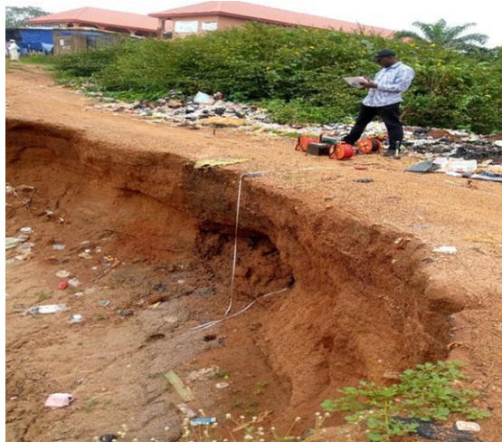
Plate 1: Geophysical Investigation at Amoyo gully erosion site in Ilorin
